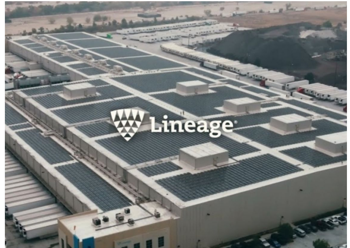
The Lineage Logistics cold storage facility in Colton, CA
